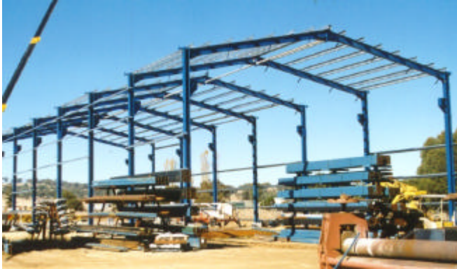
New Engineering Workshop – Sapphire City Steel and Pipe Inverell
