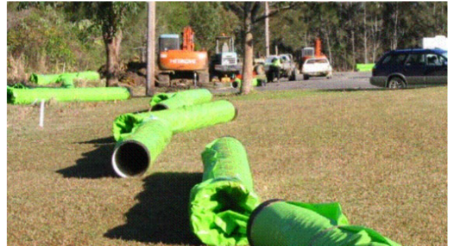
Construction of Lake Cathie Rising Main
